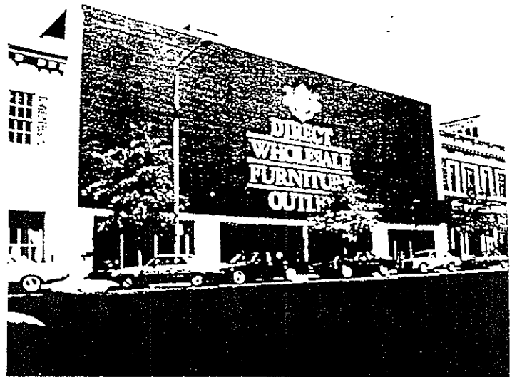
Building Inappropriately Refaced With Modern Metal Panels
